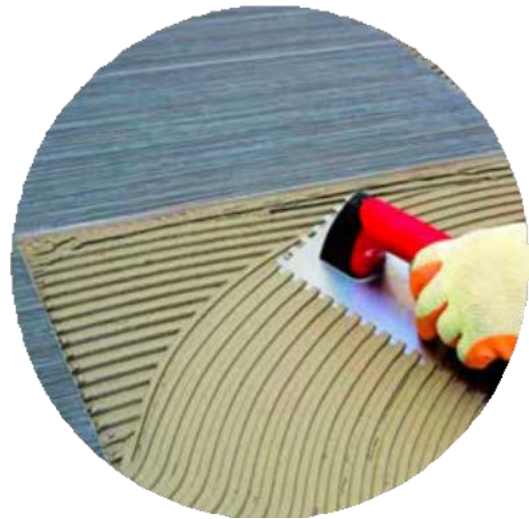
Tile and Stone Installations
