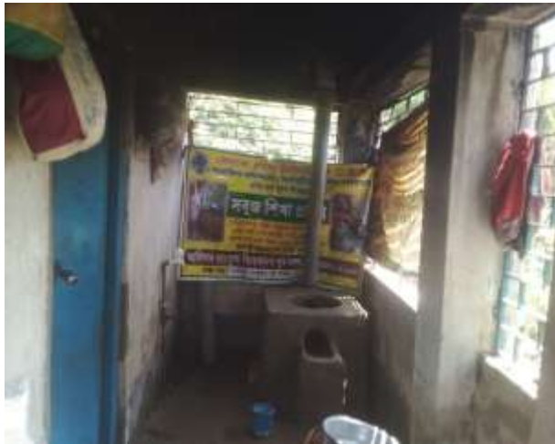
Improved Community Chullah installed at 6 ICDS Centre , Gangatikuri, East Bardhoman
