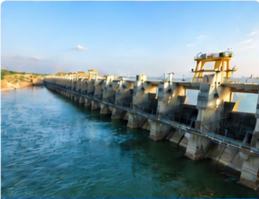
Parbati III H.E. Project (520 MW)
