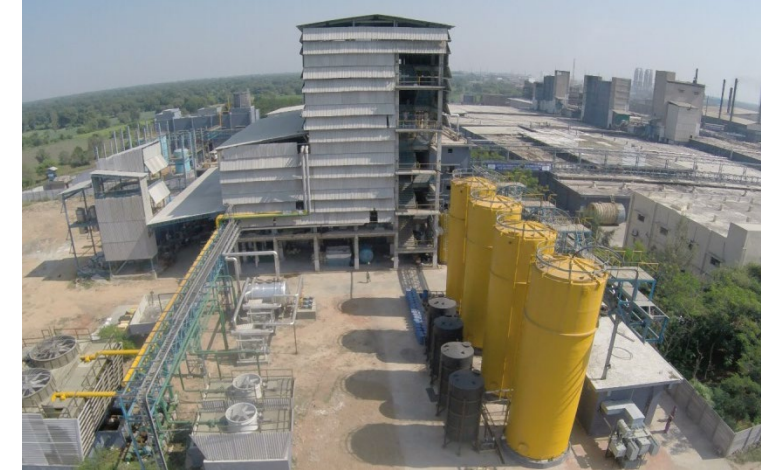
Multiple Effect Evaporator Plant (MEEP)
