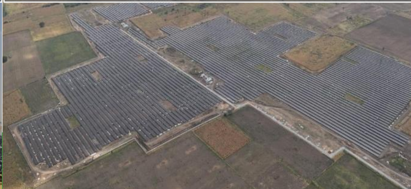
180 MWp Ground Mounted project at Tuticorin, Tamil Nadu
