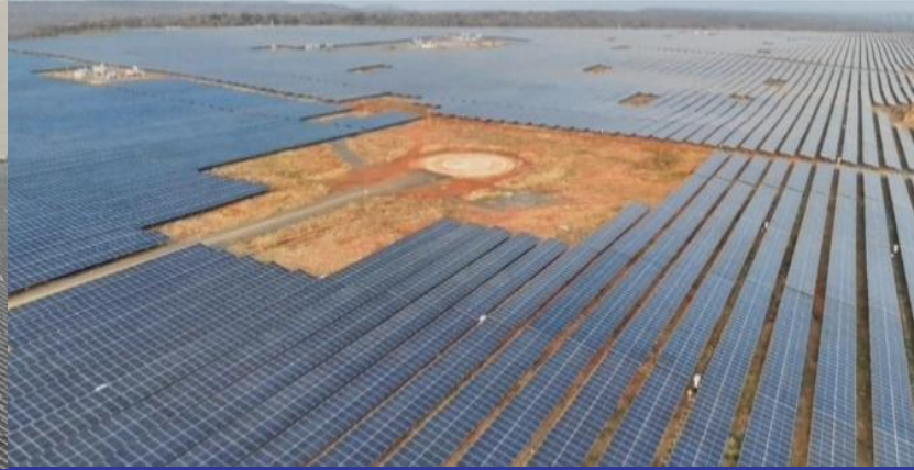
980 MWp Ground Mounted project at Kurnool, Andhra Pradesh
