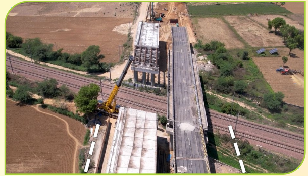
Gurgaon – Rewari Highway Project
