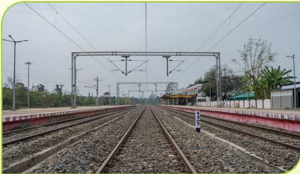
Jiribam Yard, Railway Electrification Pkg – 2
