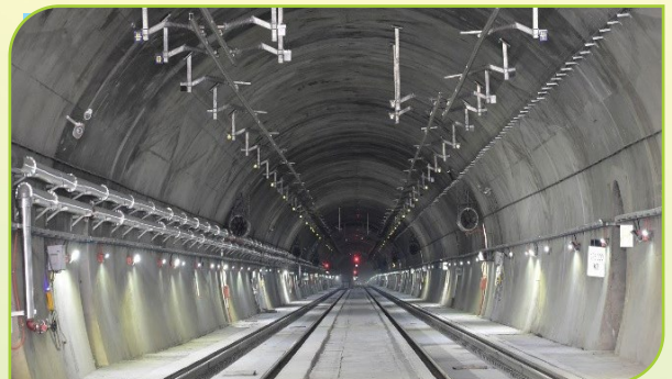
ROCS Erection in Tunnel T-50, USBRL Project
