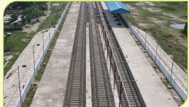
Monga Station Yard, Khulna Mongla Port Line Project, Bangladesh
