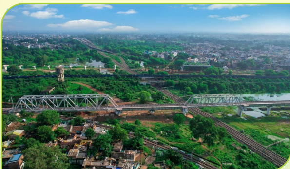
Katni Grade Separator Project
