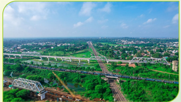
Katni Grade Separator Project
