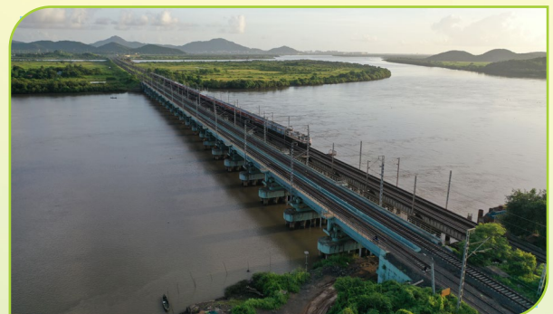
Dedicated Freight Corridor Project, CTP – 12
