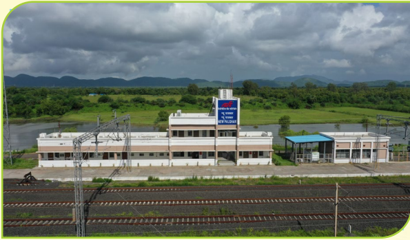
Dedicated Freight Corridor Project, CTP-12
