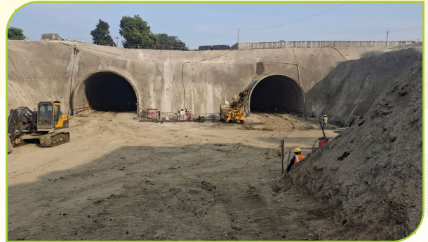
Indore Budni Tunnel T1 Project
