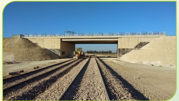
ROB above the completed double track, Algeria
