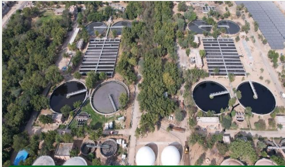
Upgradation of 100 MLD STP at Jodhpur, Rajasthan (includes solar and CBG plant)
