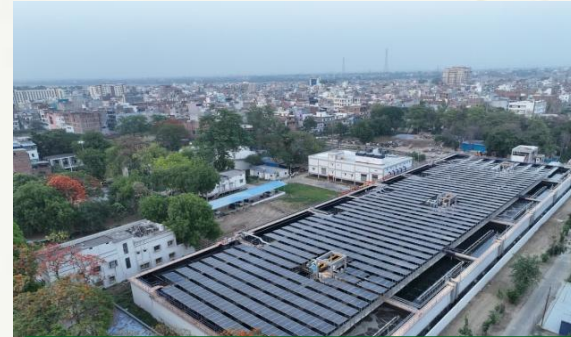
55 MLD STP, Varanasi, UP (includes solar plant)
