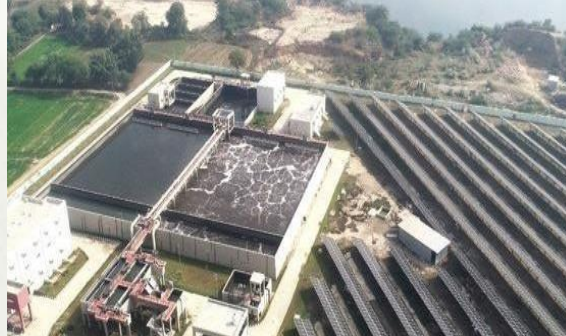
30 MLD STP Kota Rajasthan(Includes Solar Plant)
