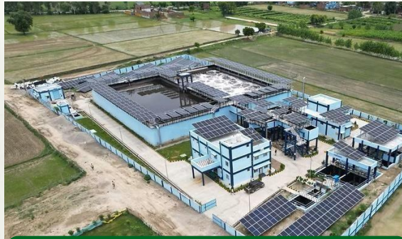
42+20+1 MLD Bareilly UP (includes solar plant)
