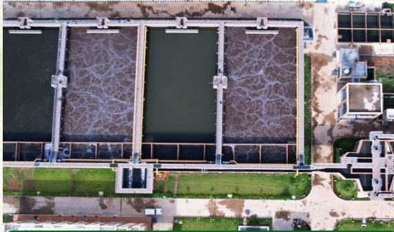
25 MLD STP, Jagdalpur, Chattisgarh
