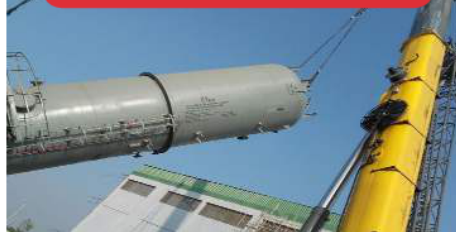
Fabrication & Erection of Equipments
