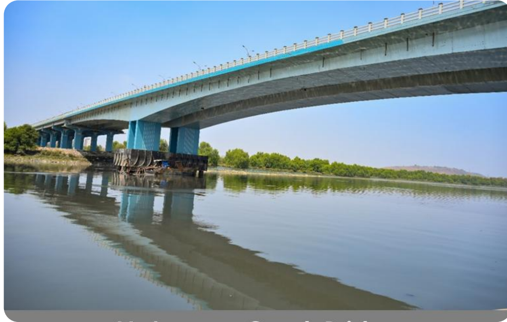
MOTAGAON CREEK BRIDGE
