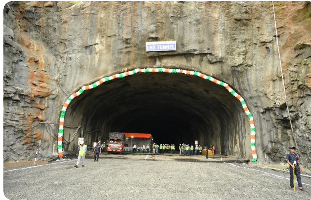
VADODARA MUMBAI EXPRESSWAY, IRCON
