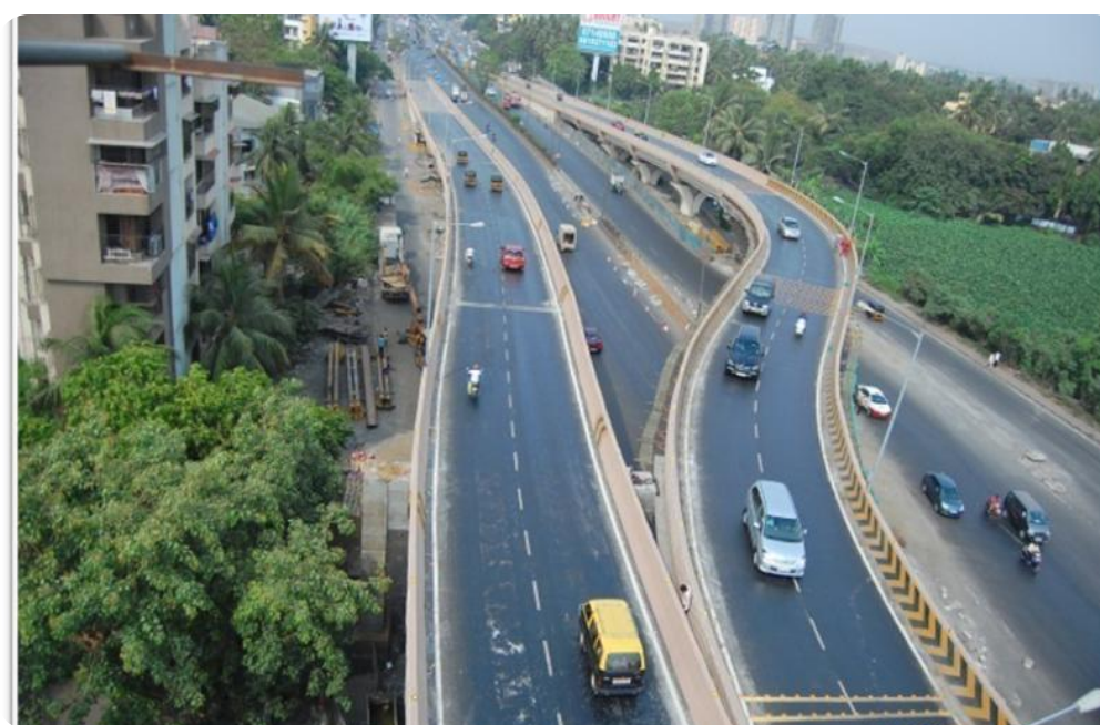
AMAR MAHAL FLYOVER
