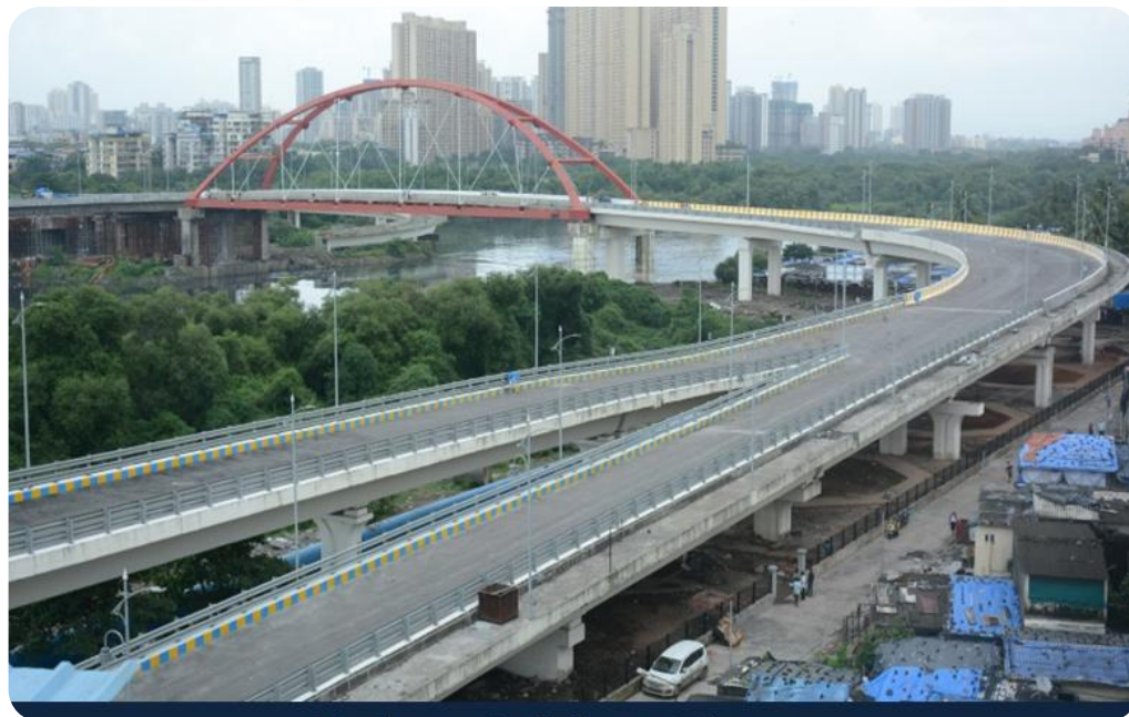
KALWA BRIDGE THANE
