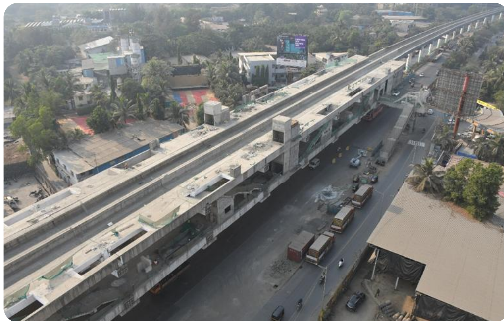
MUMBAI METRO LINE 4A
