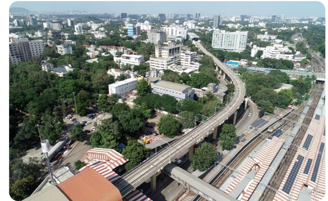
PUNE ELEVATED METRO
