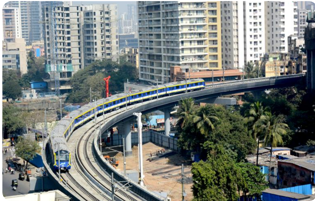
MUMBAI METRO LINE 2A
