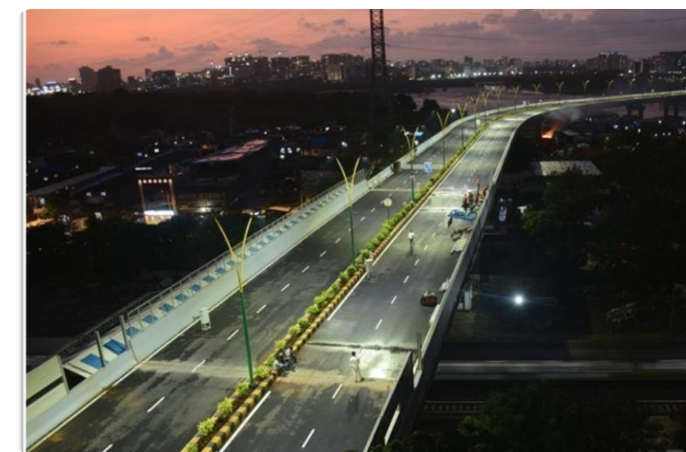
BKC- CHUNABHATTI FLYOVER
