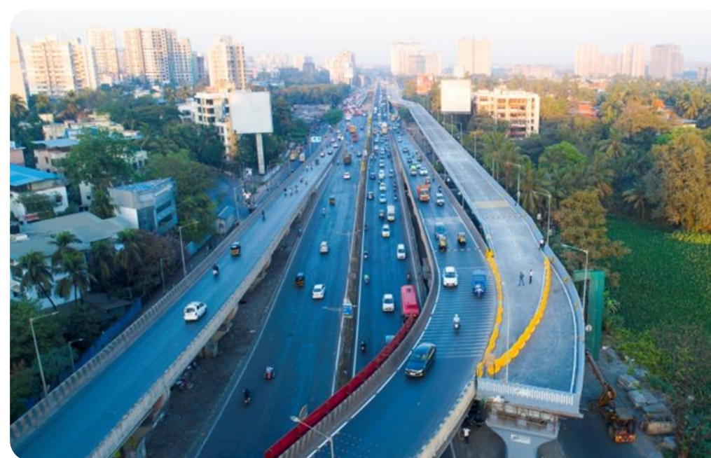
CHHEDA NAGAR FLYOVER PART 1
