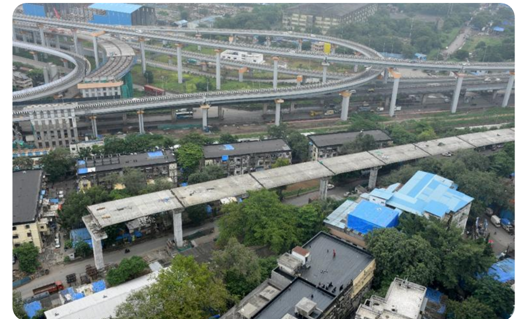
SEWRI WORLI ELEVATED
