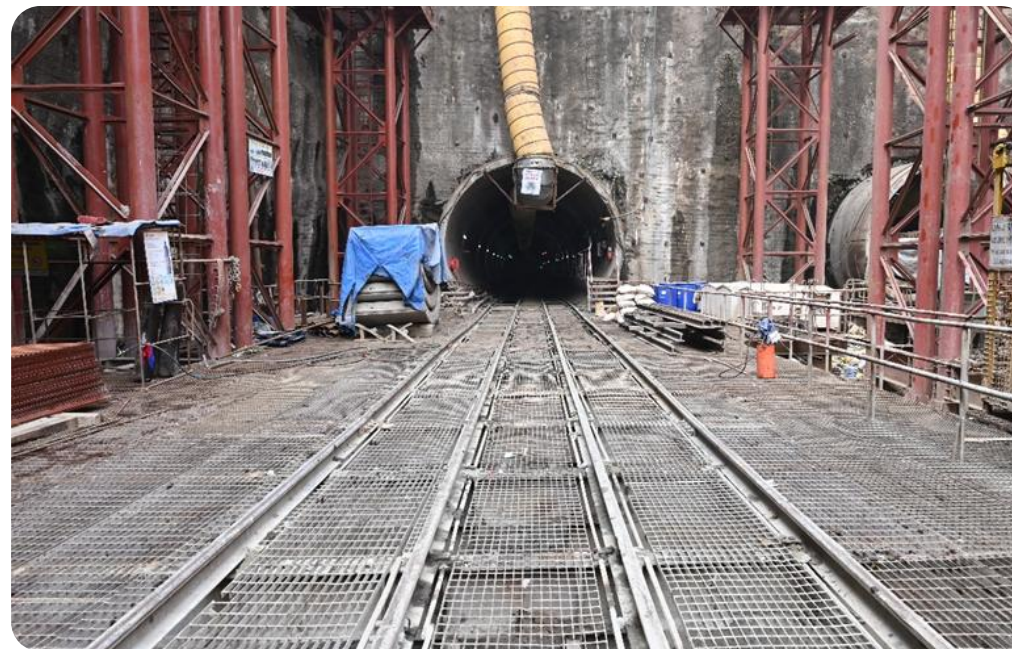
MUMBAI METRO LINE 7A
