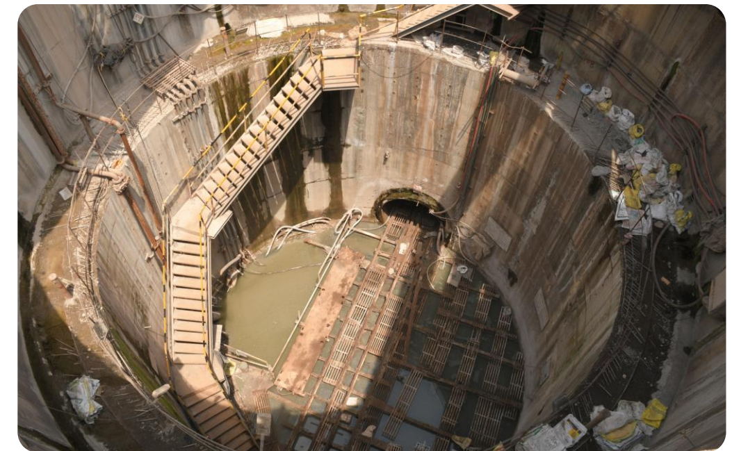
SEWERAGE PROJECT, MALAD
