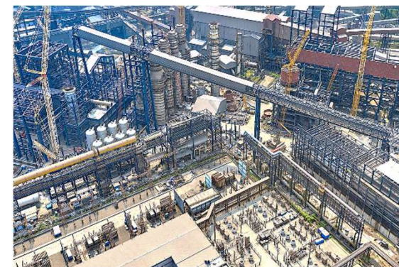
Dolvi Phase-III under construction
