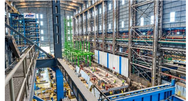
CGL-2 under construction, Khopoli
