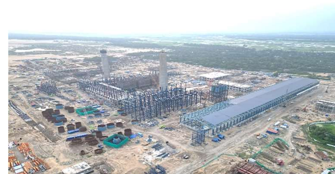
Pellet Plant under construction at JSW Utkal
