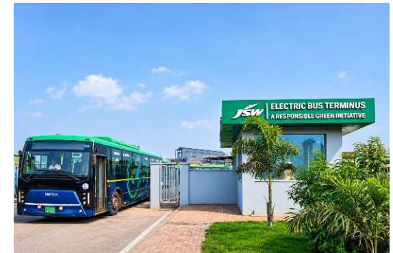
Electric Bus Terminus at Vijayanagar
