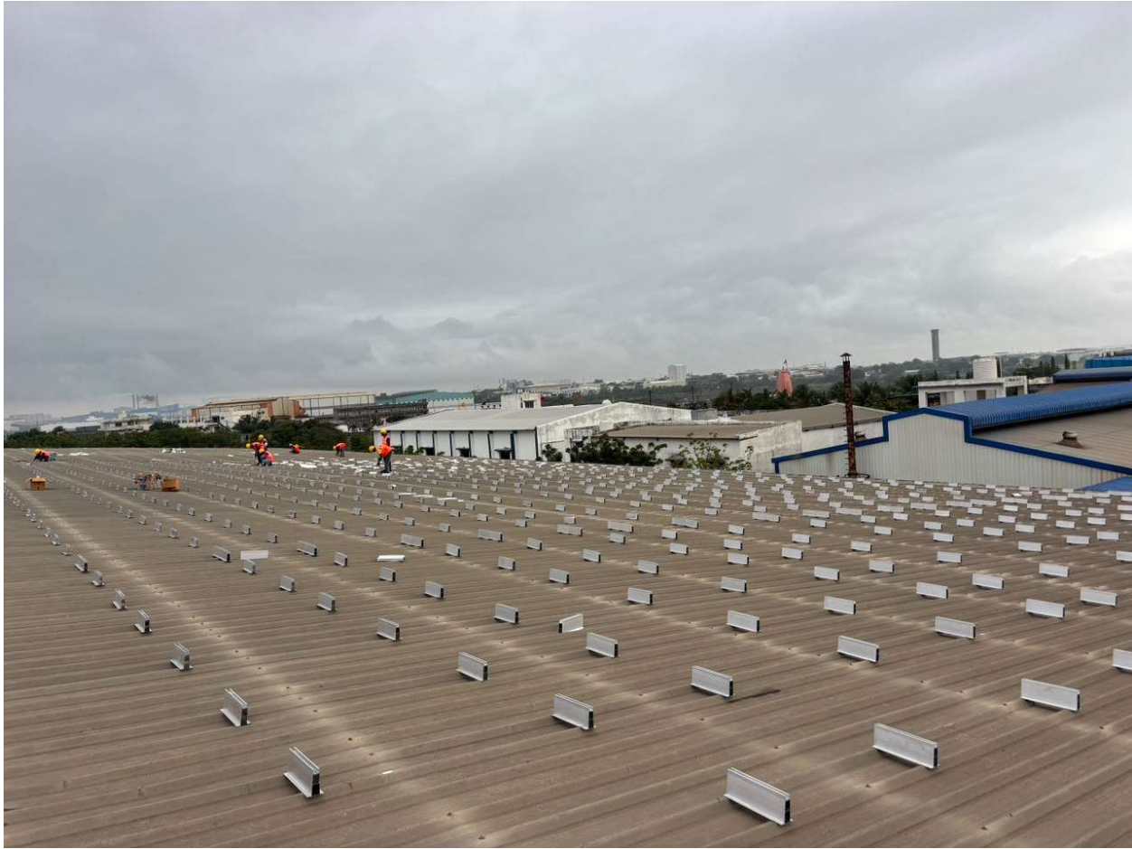
Photograph 3 - Broad rooftop view showing extensive placement / layout of mounting components across the roof and ongoing execution activity.
