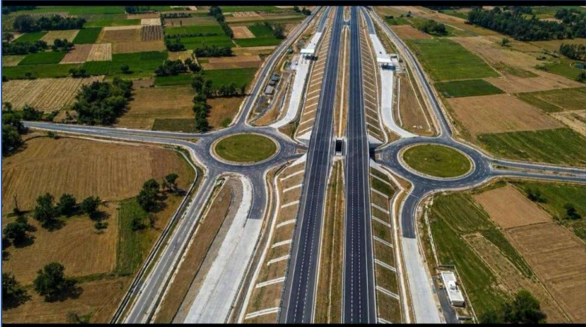
Ganga Expressway road project in Uttar Pradesh
