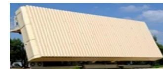
Long Range Radar TRMs, BSNs, PS
