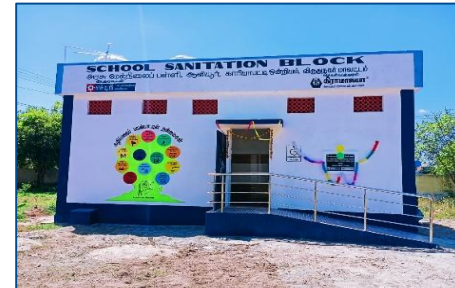
Safe Sanitation Complex, WASH
