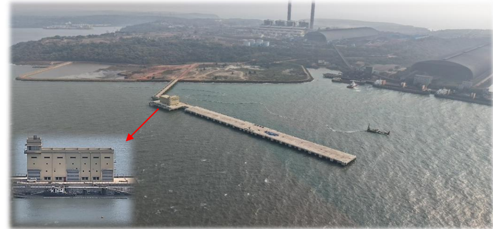
Berth and Pump house at Jaigarh
