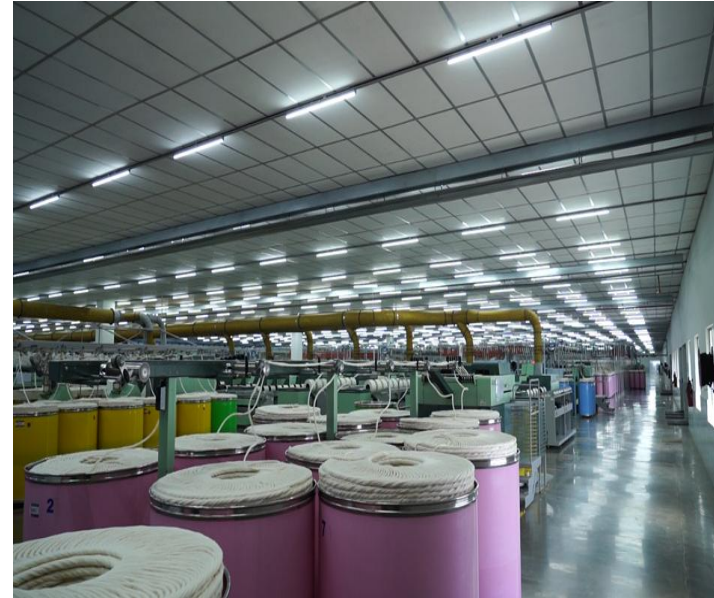
Electrification work of Spinning Mills
