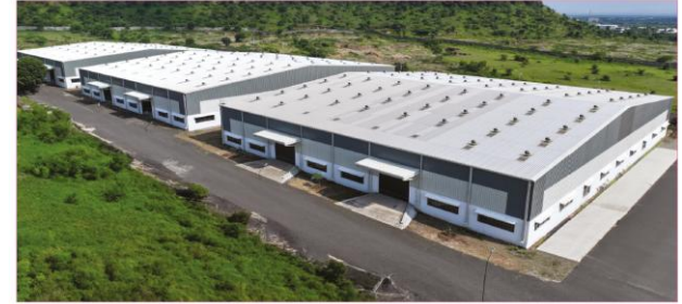
PROJECT Industrial Shed YEAR OF COMPLETION 2022 LOCATION Shendra, SEZ, Aurangabad. SPECIAL FEATURE Nearly 1,20,000 Sq. Ft. Industrial Shed with EOT crane in each bay running sidewall to sidewall for electrical panel manufacturing.
