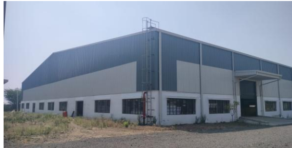
PROJECT Industrial Shed YEAR OF COMPLETION 2024 LOCATION CH.SAMBHAJINAGAR SPECIAL FEATURE - Multi Span Industrial Shed Of 80, 000 Sq.Ft at Ch.Sambhajinagar
