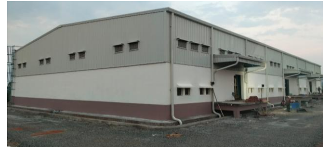
PROJECT Warehouse YEAR OF COMPLETION 2025 LOCATION KOLHAPUR SPECIAL FEATURE - Construction Of 3000 MT Capacity Pre-engineered Building Warehouse With Ancillary Workshop Belewadi Tal: KAGAL, Dist: Kolhapur
