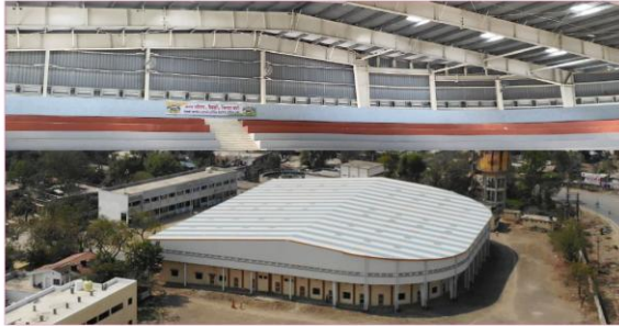
PROJECT Indoor Stadium YEAR OF COMPLETION 2016 LOCATION Deoli, Wardha SPECIAL FEATURE Clear Span Structure of 62m, with complete civil works and seating capacity of 3,000 peoples.
