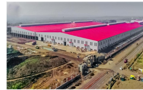
Pre-engineered Steel Buildings
