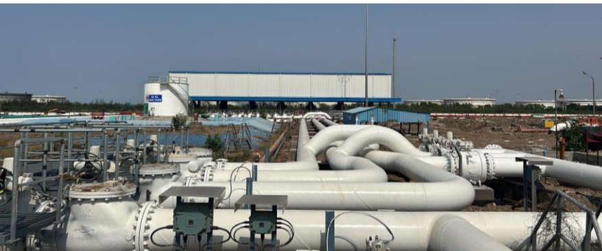
Booster to Blending Unit Piping works at Vadinar, Gujarat
