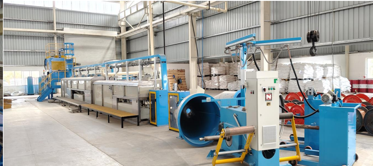
Elastomeric cables facility at Vadodara, Gujarat
