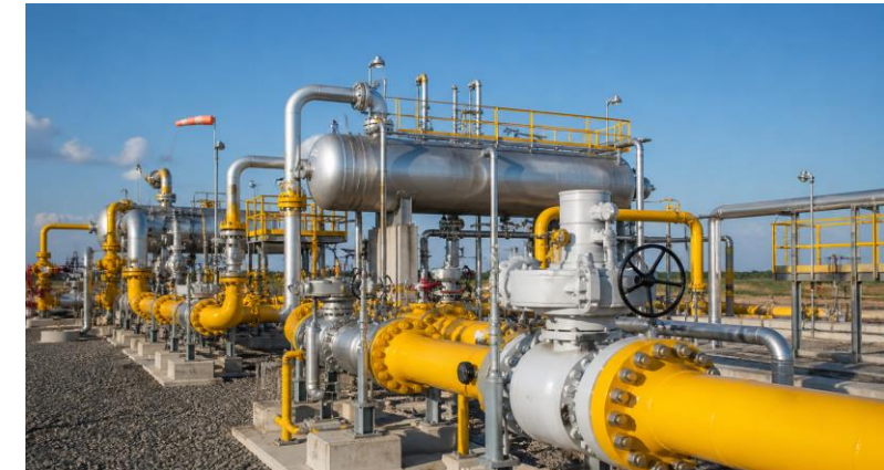
International - Composite Station Works (Oil & Gas)
