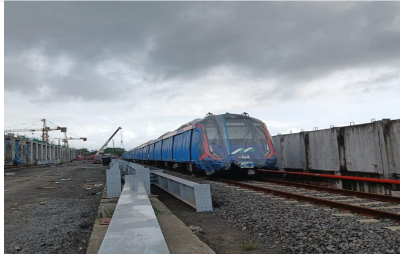
Track works, Mumbai Metro
