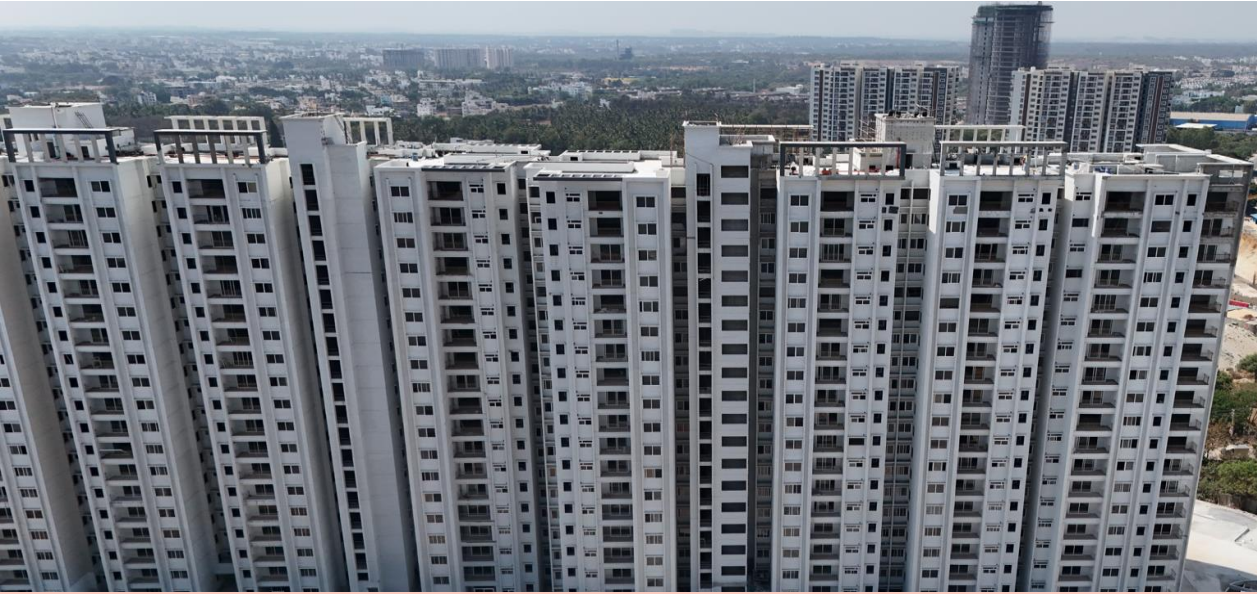
High Rise Residential Building, Bangalore, Karnataka
