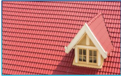
Domestic Roofing & Cladding
