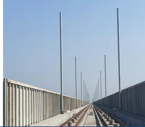
Supply of electric masts for bullet train project in India
