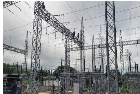
138kV Substation and Transmission Line Project in Nicaragua
