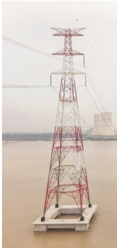
400kV D/C Rooppur-Gopalganj Transmission Line, Bangladesh
