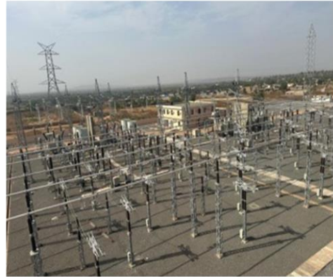
225/30 kV Substation project at Mali
