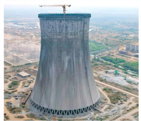
Cooling tower at Udangudi and Yadadiri
