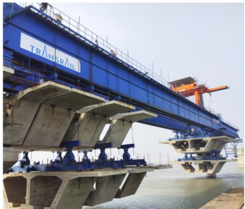
10.2 km long Road Bridge over river Kosi (Bihar)
