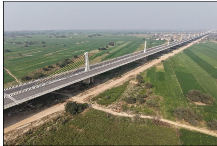
L&T Daewoo- Patna Bridge
