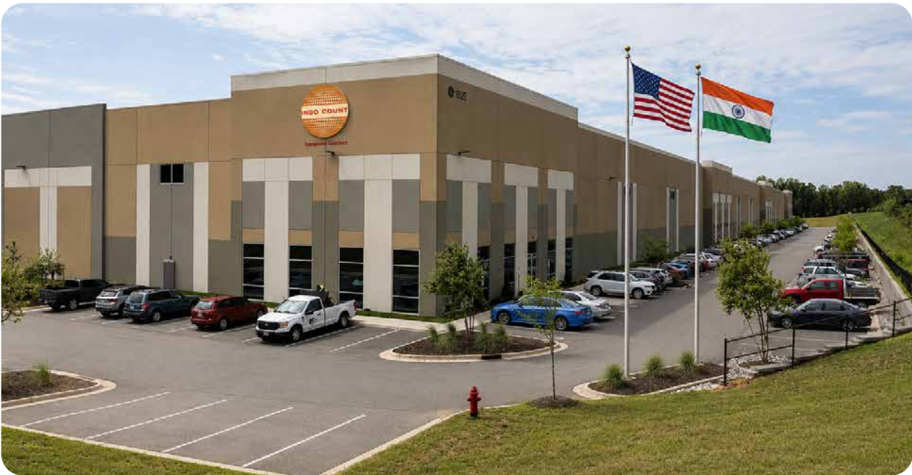
INDO COUNT GLOBAL EAST, INC. KERNERSVILLE (North Carolina) This greenfield manufacturing facility, newly commissioned in 2026, drastically scaled Indo Count's utility bedding footprint, adding a massive production capacity of 18 million pillows annually to directly serve the United States market.
