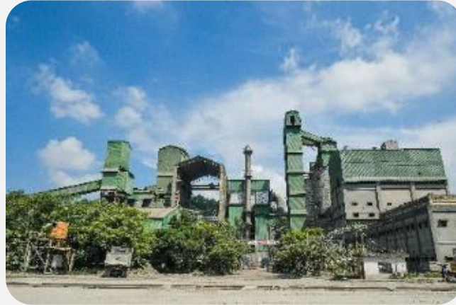
Guwahati Grinding Unit
