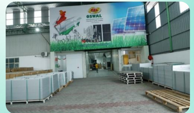
Facility for manufacturing solar modules
