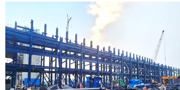
Utkal Pellet Plant: Induration Building Construction in Progress
