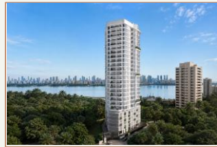
RUSTOMJEE CLIFF TOWER, MOUNT MARY, BANDRA-W
