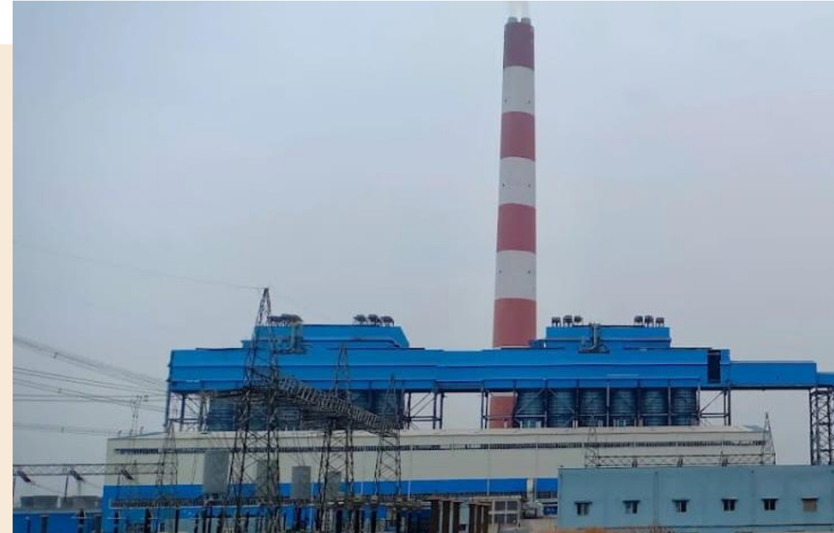
Actual site photo of 2x300 MW SKS Power Plant
