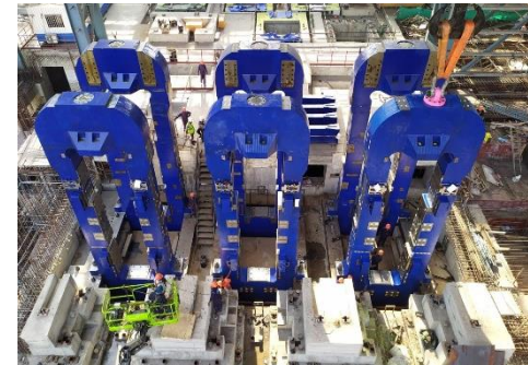
Dolvi Phase-III: Roughing Mill Housing erected
