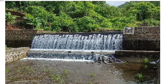
Check Dam in Vijayanagar
