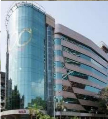
Saraswat Bank Bhavan Phase I : Upto 7 th floor
