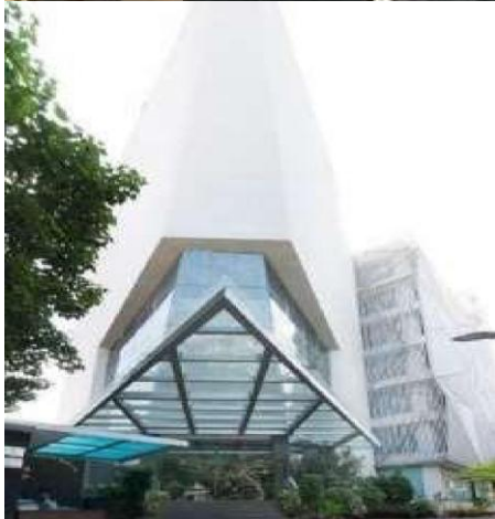
CCIL Bhavan Phase I Upto 6 th floor
