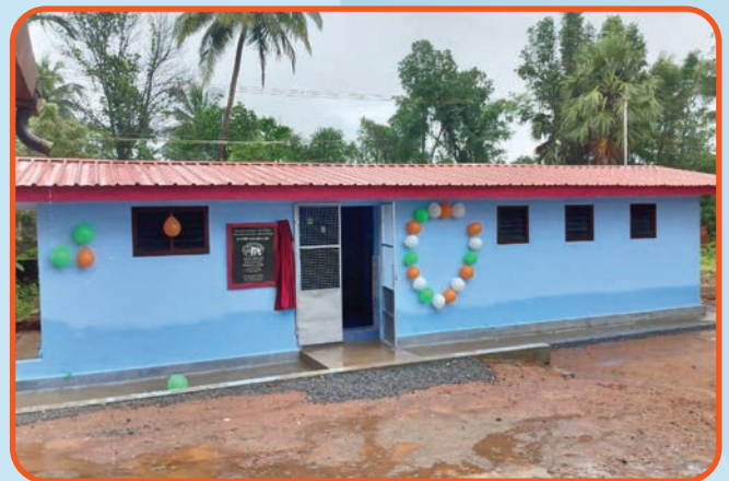
Repair and Renovation of Toilet at the Govt. Girls School, Bangady, Karnataka
