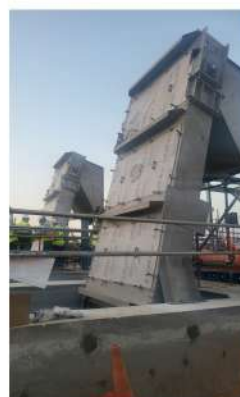
Twin Belt Conveyor with Deflector Plate Assembly, Jet Breaker, MM 2 MM Mechanical Coarse Screen
