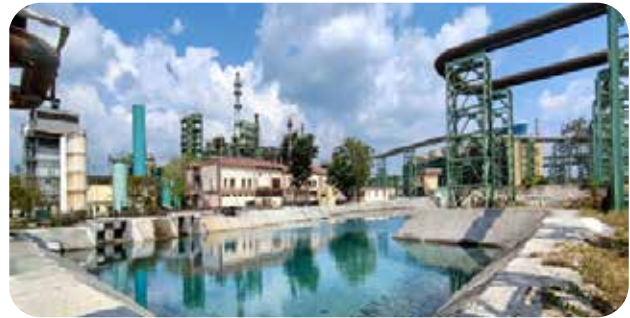
New Storm Water pond at Ref-I/II area
