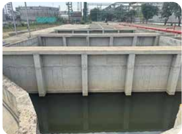
Oil catchers in New Storm Water ponds
