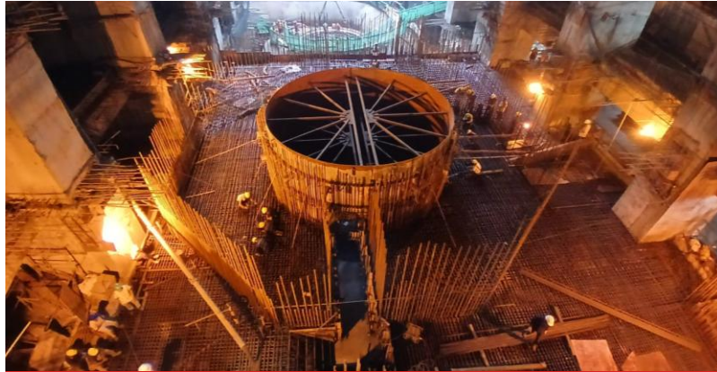
Commencement of concreting works for Unit 7 at EL 102.25m
