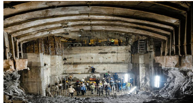
Completion of Interdependent Milestone (IM-1), marked by the handover of Draft Tube Unit-1 to the E&M Agency.
