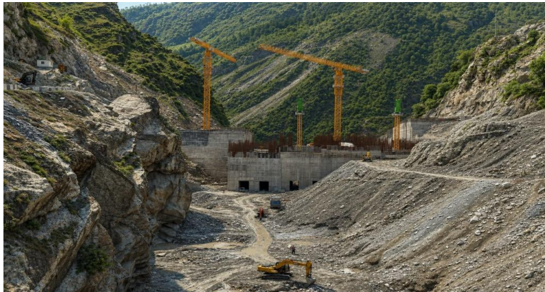
Achieved 50% dam concreting milestone with 32,000 CuM poured in April 2026.
