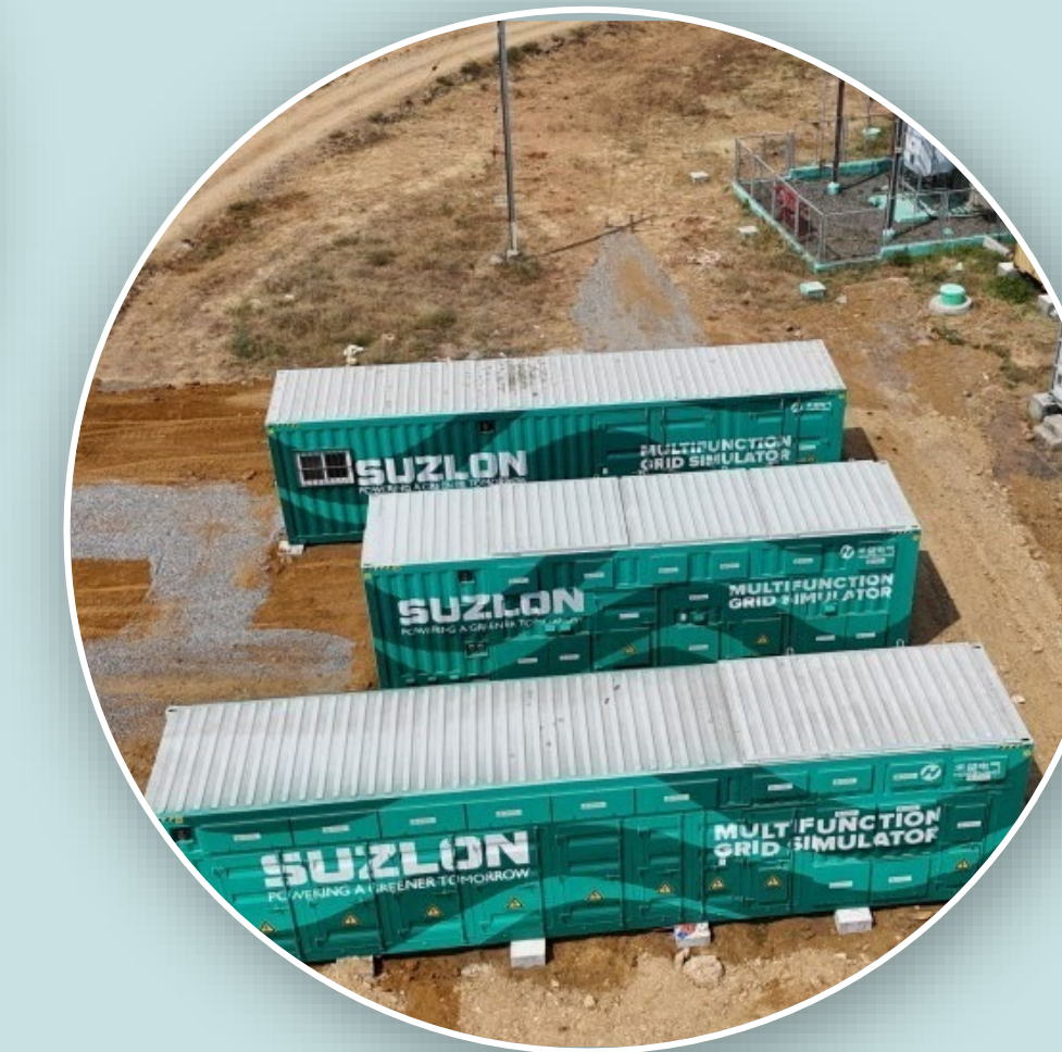
Grid Compliance testing at prototype site
