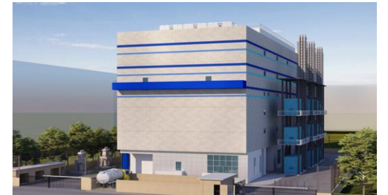
DATA CENTER BUILDING
