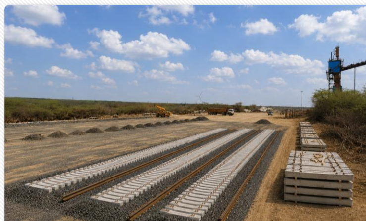
Railway Siding – Earth Work Completed, Ballast Laying and Sleeper Laying Work in Progress
