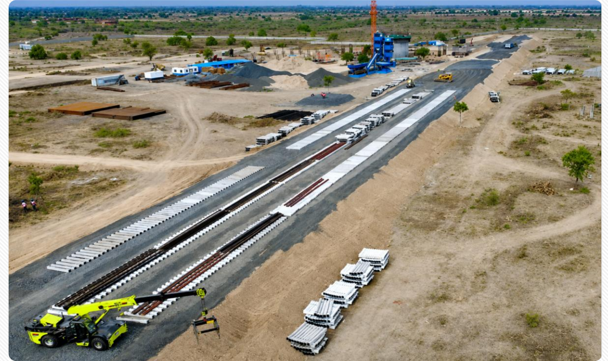
Railway Siding – Track Laying in Progress
