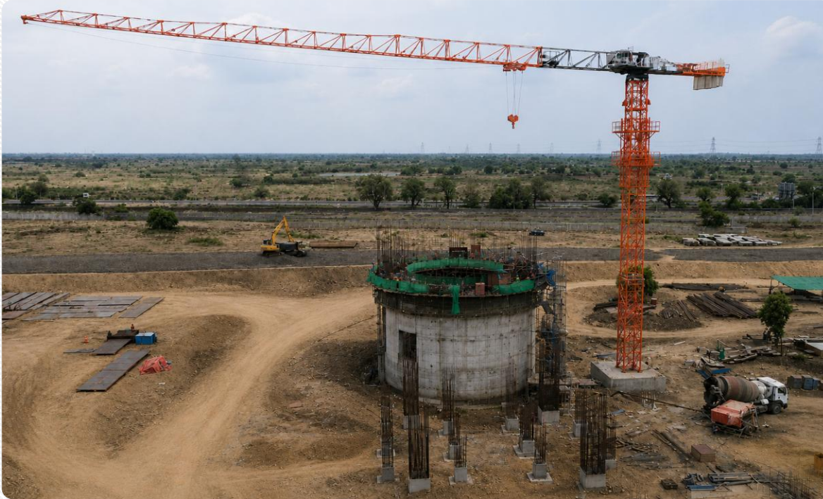
Silo Casting Work in Progress
