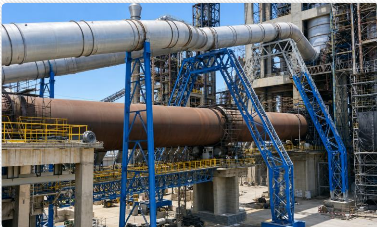
Kiln Rotation is Complete, Ready for Brick Lining
