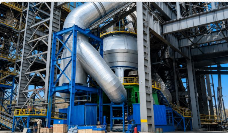
Raw Mill – Mill and Gearbox Overhaul is Complete
