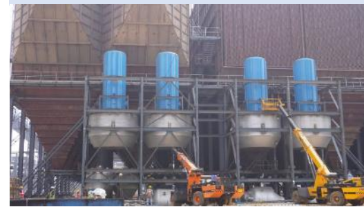
Induced Draft Cooling Tower
