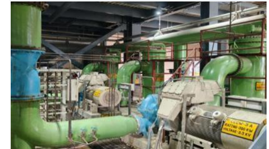
Circulating Water Motor Erection
