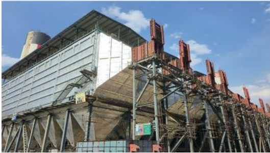
Induced Draft Cooling Tower
