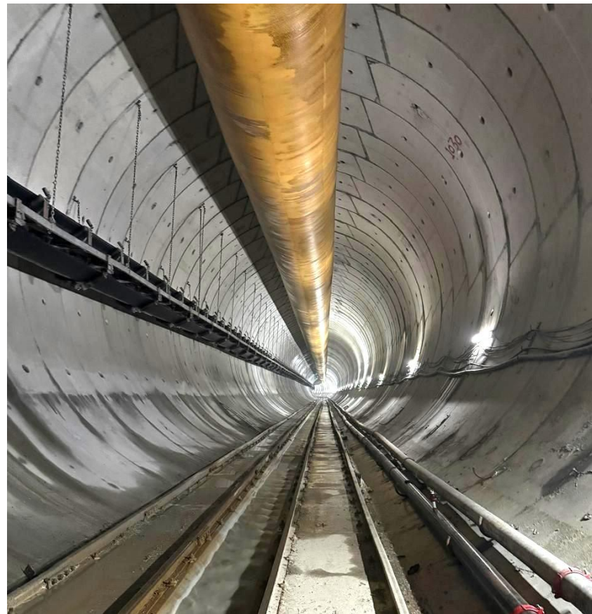
Head Race Tunnel
