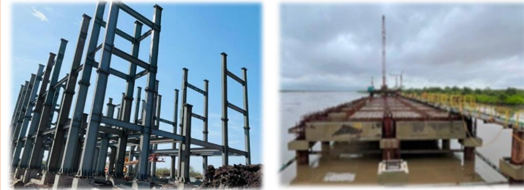
Expansion work at Dharamtar Port
