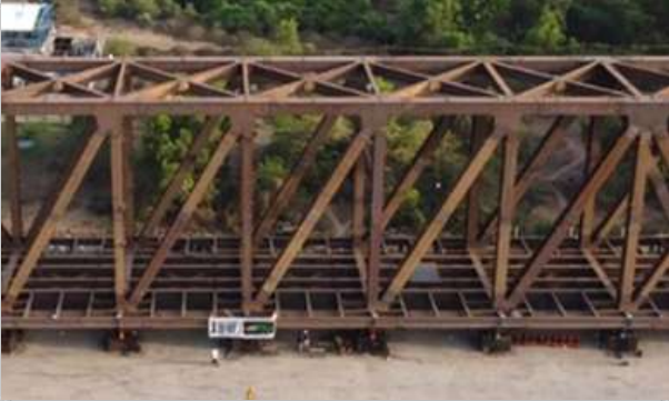
Steel Bridge Structures
