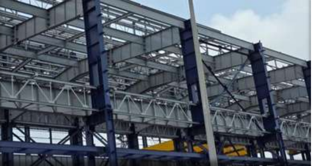
Erected Structure Of AMNS
