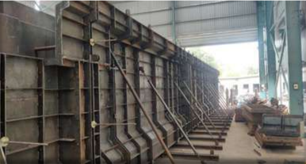
Pier Shutter – L&T
