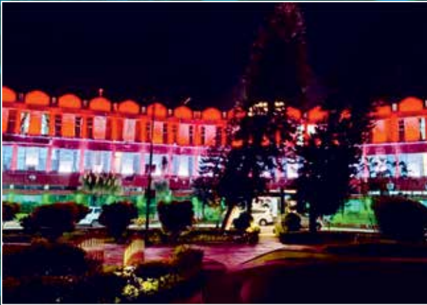
Malda DRB Building, West Bengal
