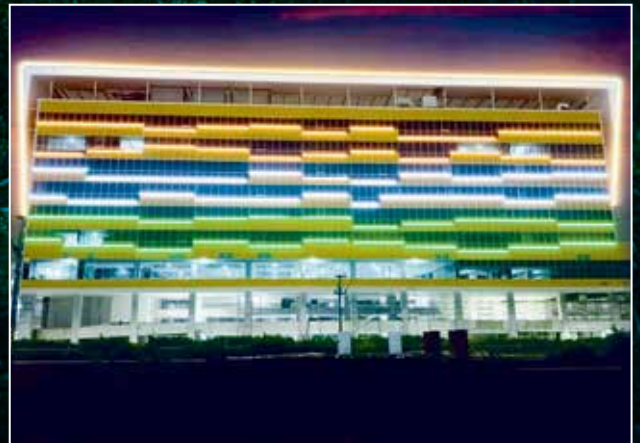
Sabarmati Bullet Train Terminal, Ahmedabad
