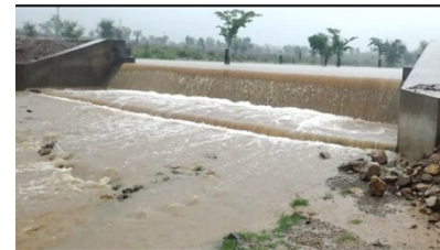
Water Conservation Project
