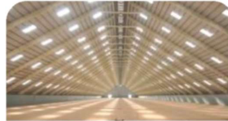
Approx 90,000 sq. m. 'A' frame structure with a centre height of 42 metres and clean span of 84 metres specially designed for the sugar storage requirements for a major Indian sugar company in Kandla, Gujarat
