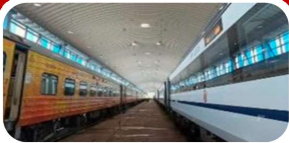
Vande Bharat Mumbai Central Pit Line Shed
