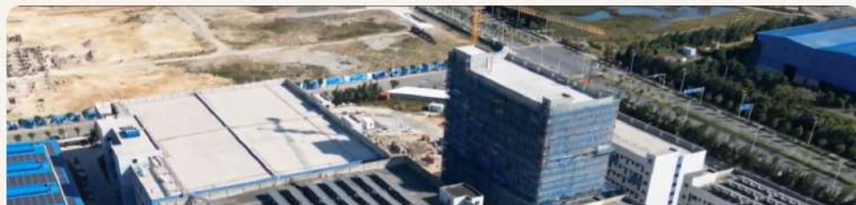
NEW INTEGRATED MANUFACTURING FACILITY · WEST BENGAL · UNDER CONSTRUCTION 2026
