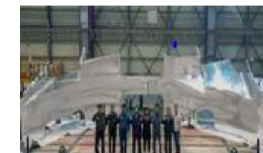
Thermal shield repair ITER Project
