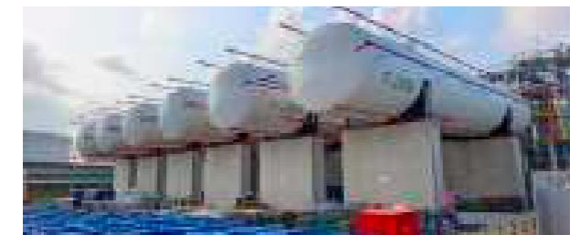
Hydrogen tank installation
