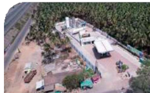
LNG/LCNG fuel stations
