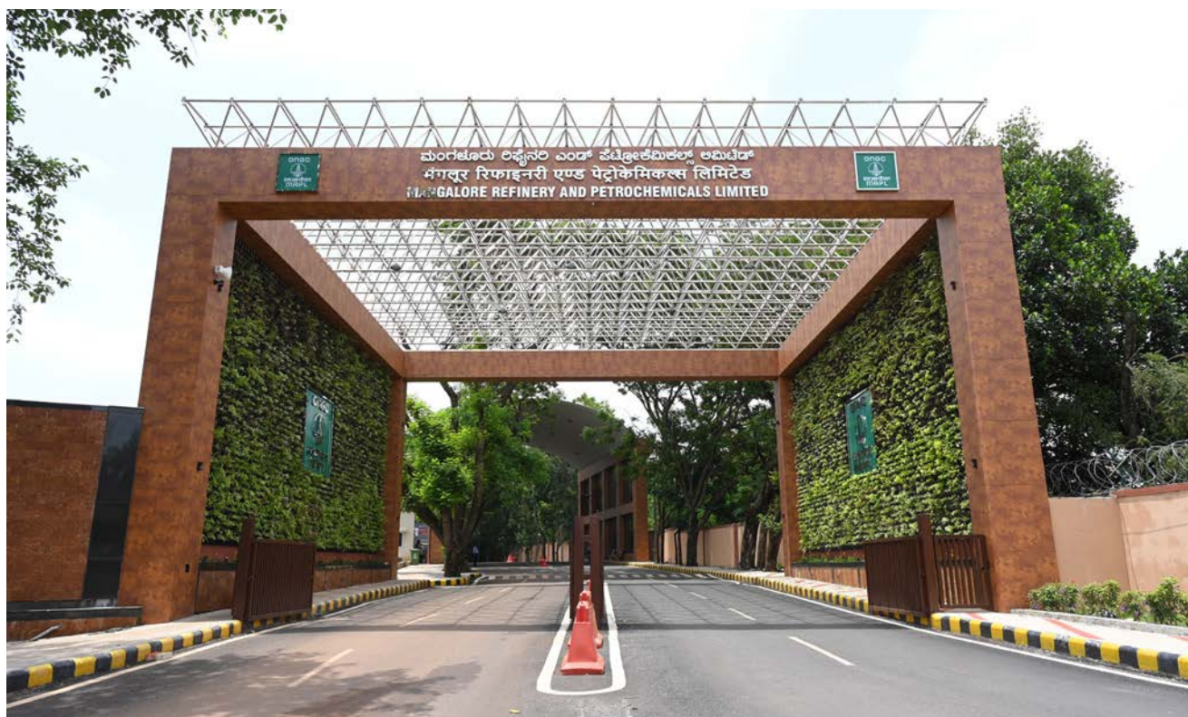
Refinery Complex Entrance
