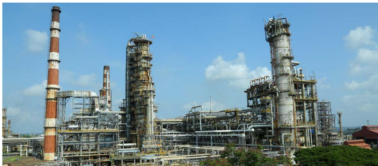
Crude Distillation Unit - Phase 2
