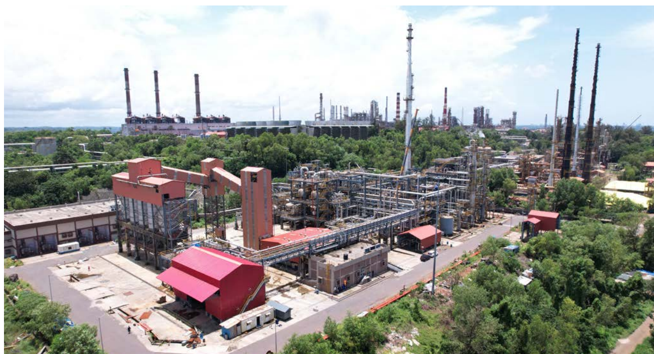
Sulphur Recovery Unit
