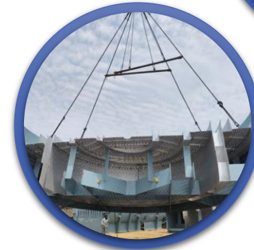
Project Cargo Execution (3,500 CBMs)
