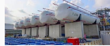
Hydrogen tank installation
