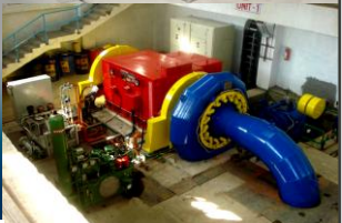
Hydro Turbine Generator & Site Installation
