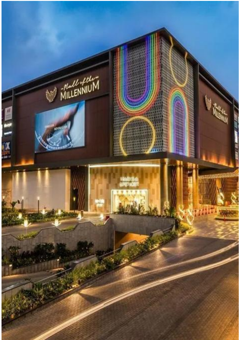
Marketcity Mall ~27 lac sq. ft Phoenix Marketcity, Pune 2 B + 6 Floors + MLCP of 10 Levels
