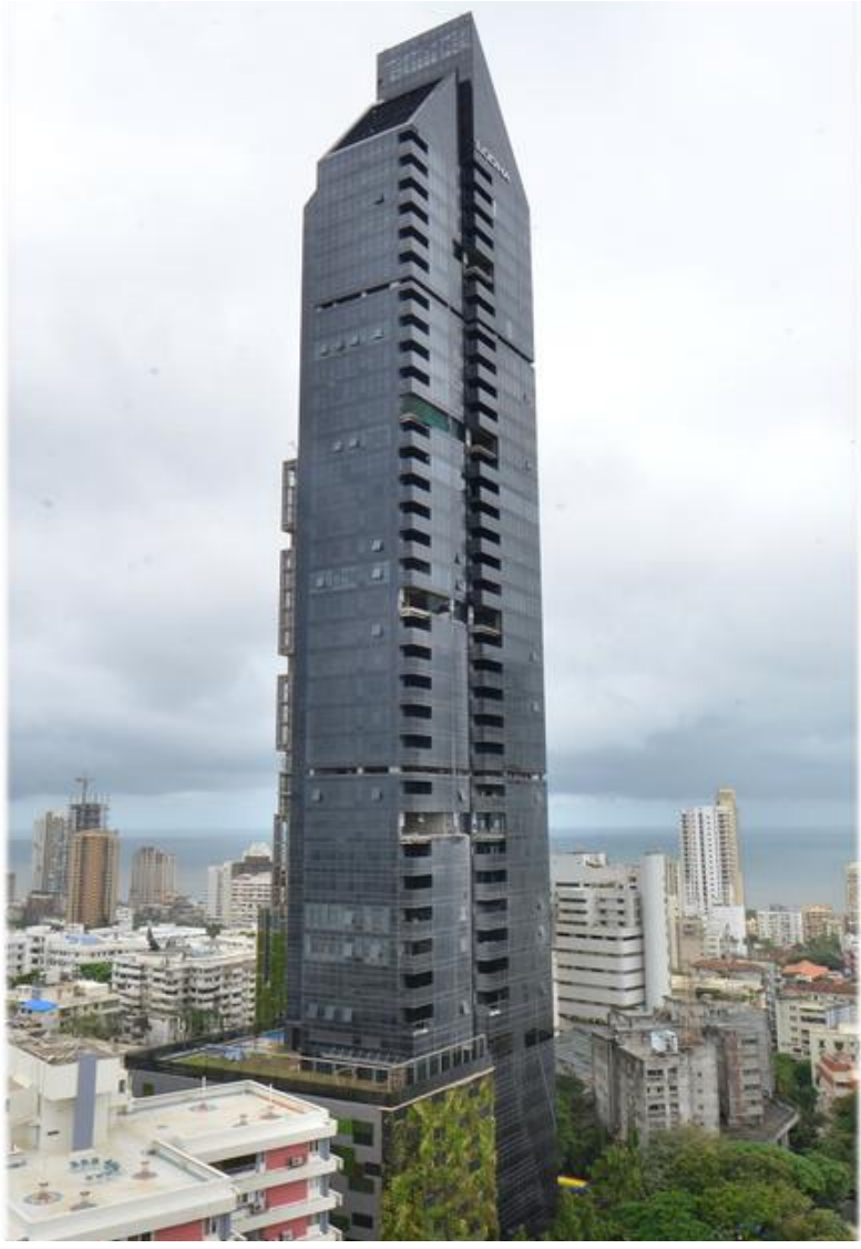
One Altamount ~206 Meters; ~4 lac sq. ft Lodha Group, MMR India's Tallest Composite Residential Tower 3B + GF + 43 Floors + Crown
