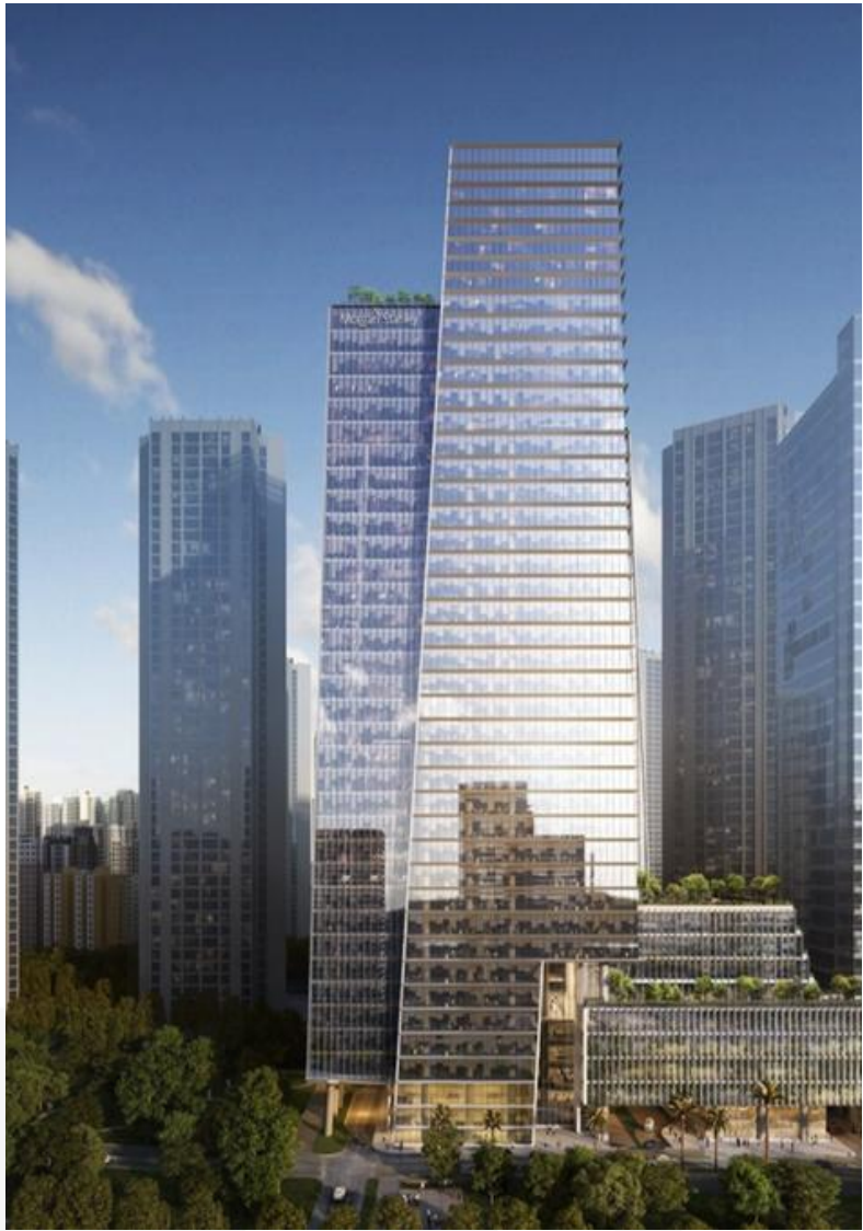
ALTIMUS COMMERCIAL TOWER ~17 lac sq. ft K Raheja COrp 1B+GF+8P+1A+33 Office Levels+2 SF
